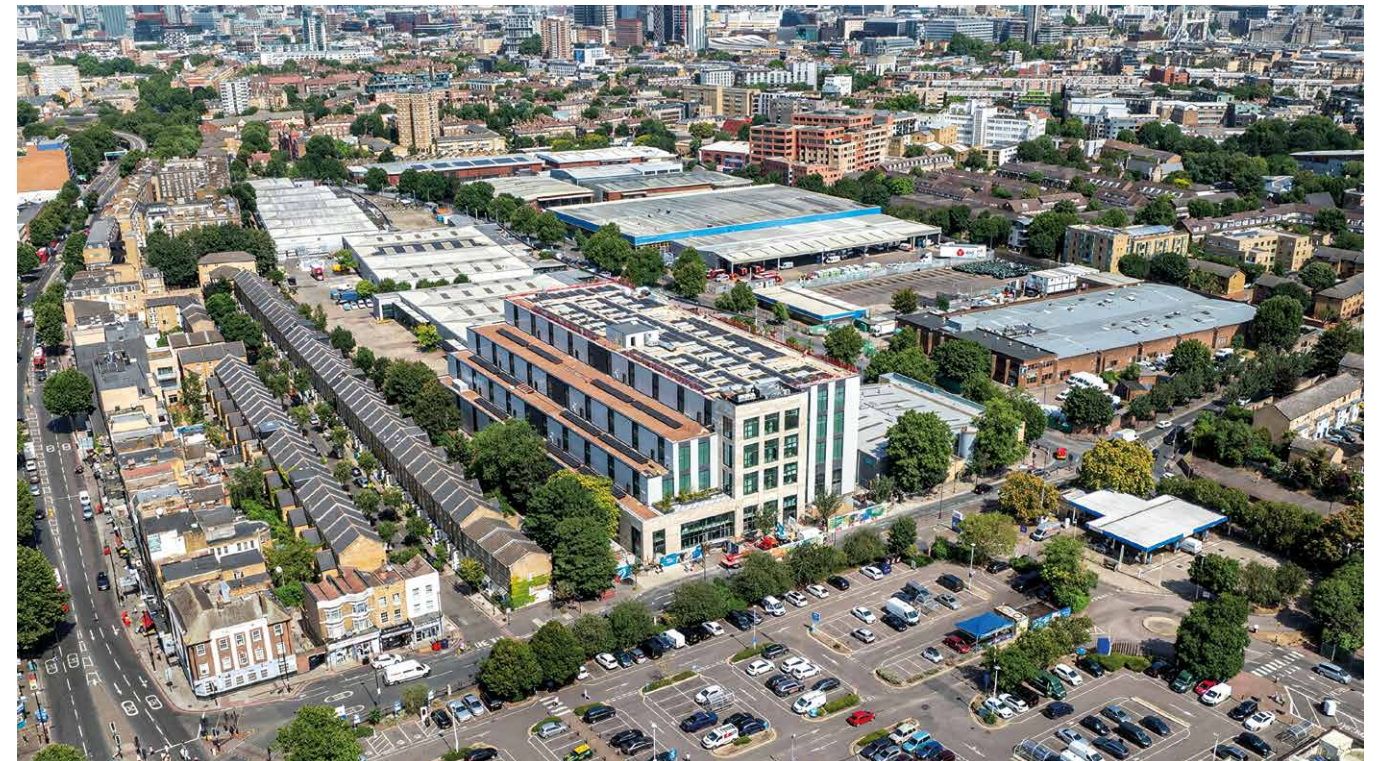
Projektfoto: Southwark Urban Logistics, © British Land / Architektur: The Harris Partnership
